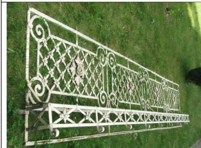
Figure 35 – balcony balustrade cut for sandblasting
