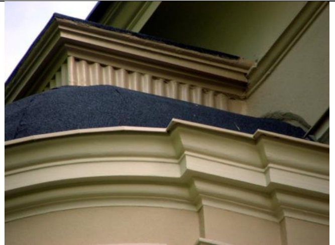
Figure 6 – a felted roofing of the corner annex
