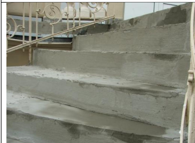
Figure 53 – the first layer of insulation against water on the terrace stairs
