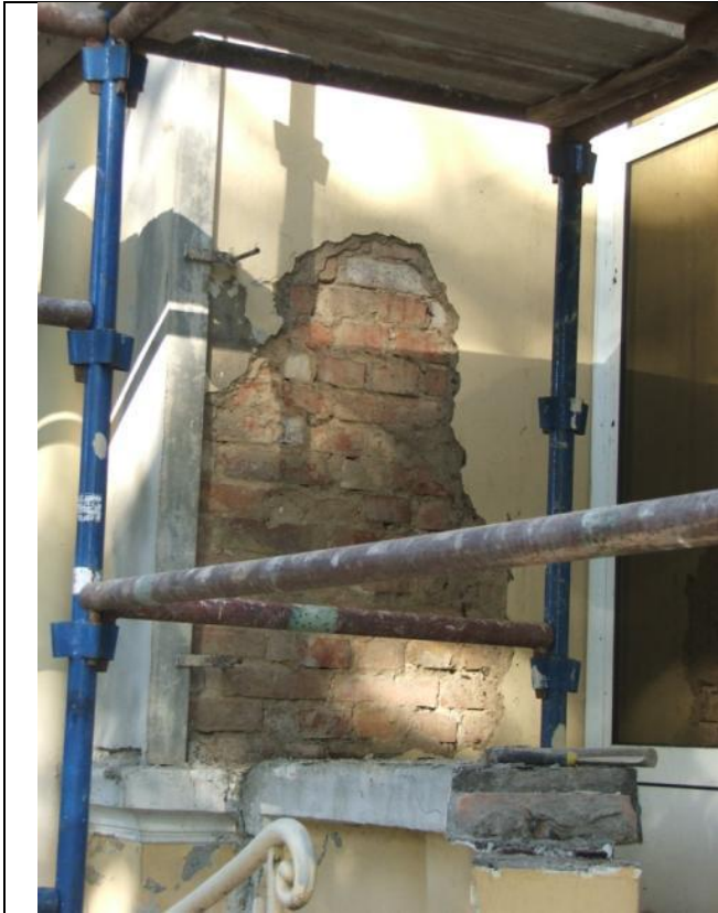
Figure 31 – the east wall, hacking the bad plaster off
