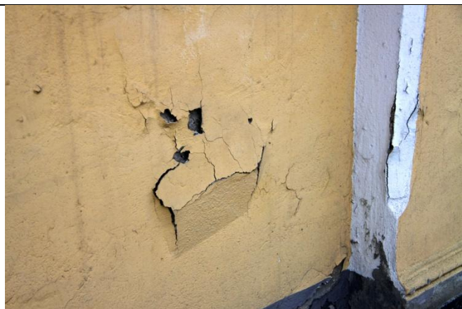
Figure 9. condition of the plaster
