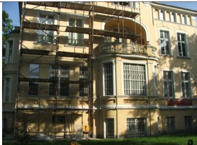
Figure 12 – (21.05.2014) Setting up the scaffolding along the west wall of the school building
