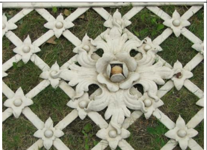
Figure 36 – part of balcony balustrade suffering from corrosion
