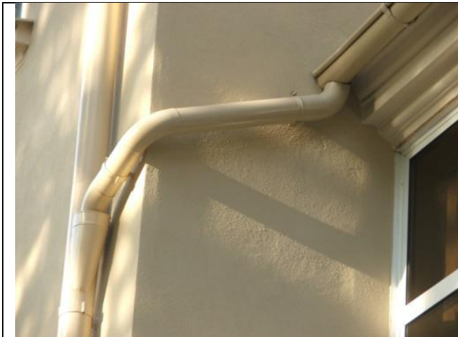
Figure 41 – flumes on the east wall of the building
