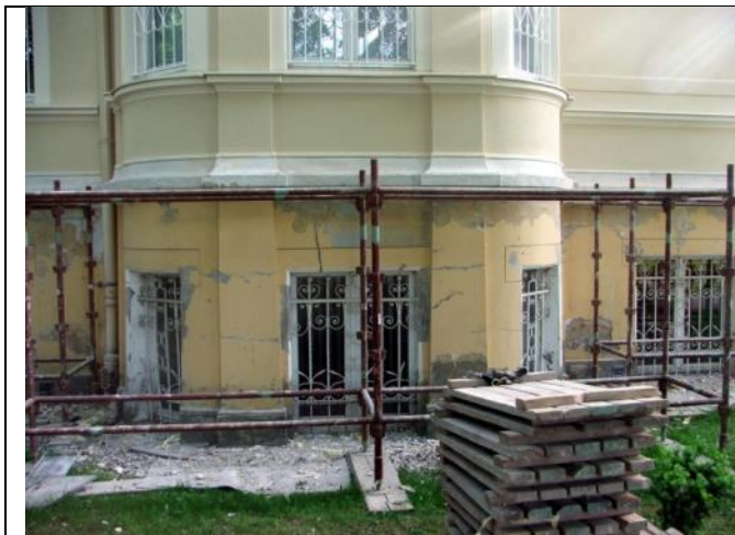
Figure 11– the base course of the building before renovation
