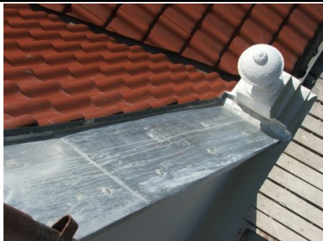
Figure 13 - plating coping with tinplate
