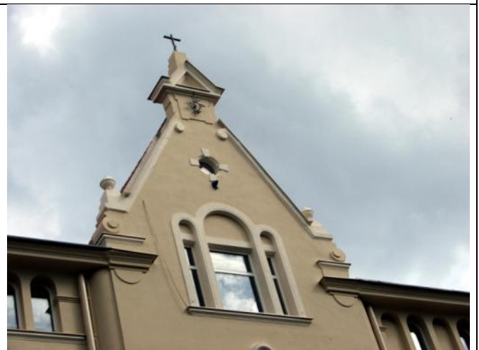
Figure 24 – coping on the west wall of the building
