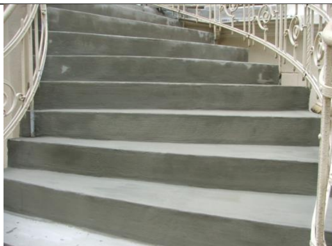
Figure 54 – the second layer of insulation against water on the terrace stairs
