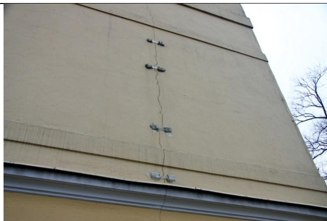
Figure 10. the wall began to crack
