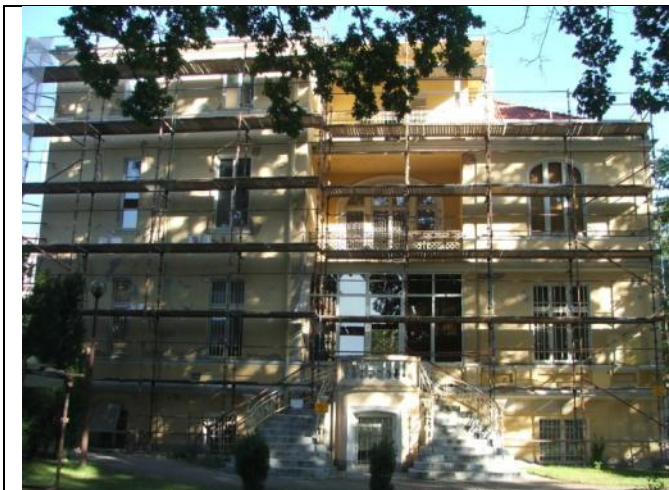
Figure 27 – Setting up the scaffolding by the east wall of the school building (23.06.2014)
