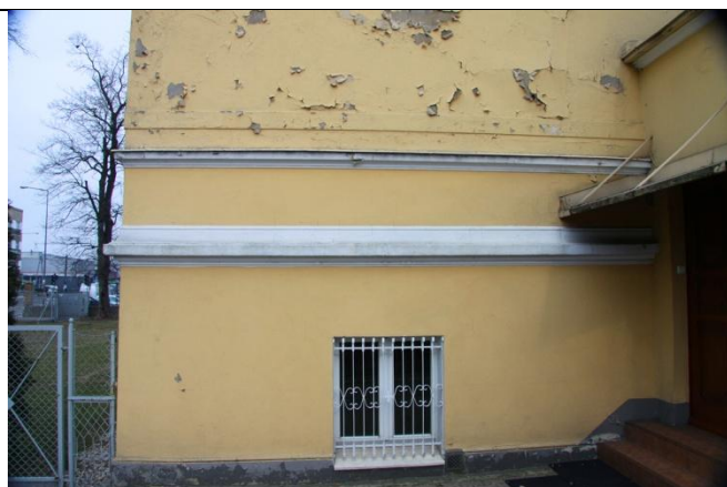
Figure 3. condition of the plaster
