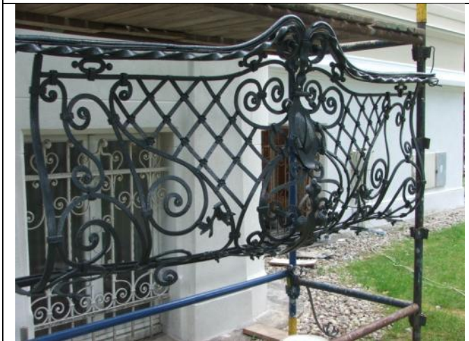
Figure 19 – balustrade of the balcony after sandblasting and painting
