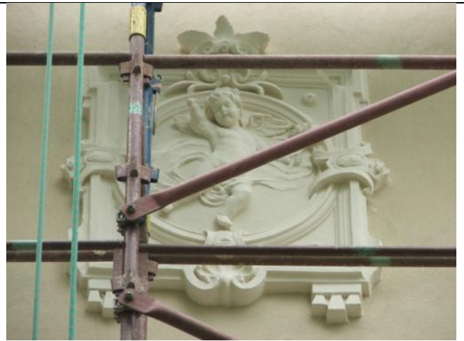
Figure 8 - the molding after the repair work
