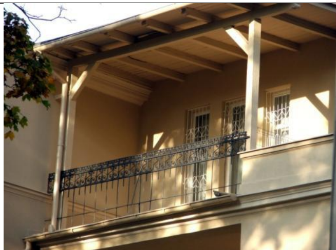
Figure 40 - balcony balustrade after sandblasting and painting – on the 2 nd floor
