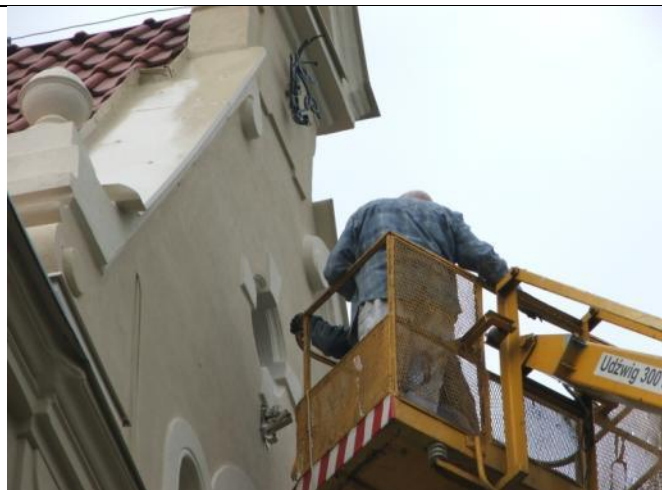
Figure 28 – painting decoration details and removing old flag handles on the west wall of the building - recommended by inspector in charge of the renovation (24.06.2014)
