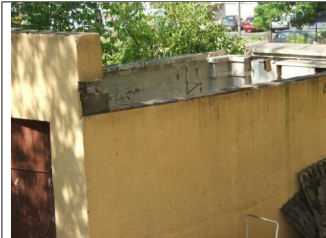
Figure 51 – renovation of garage – removing the roof
