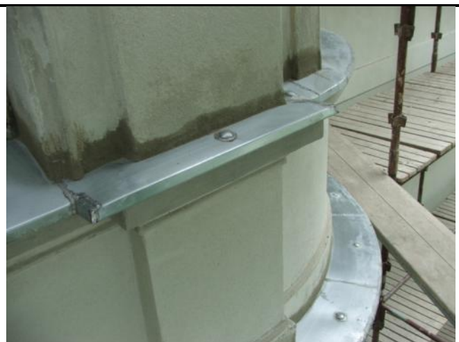
Figure 4 – plating cornices with tinplate
