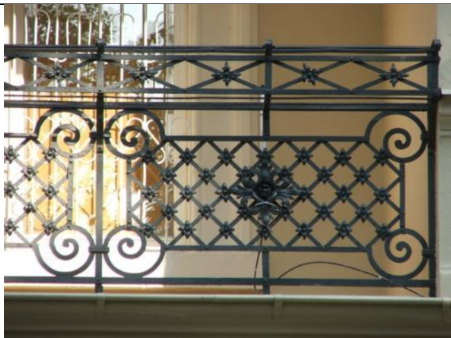
Figure 39 - balcony balustrade after sandblasting and painting – on the 1 st floor
